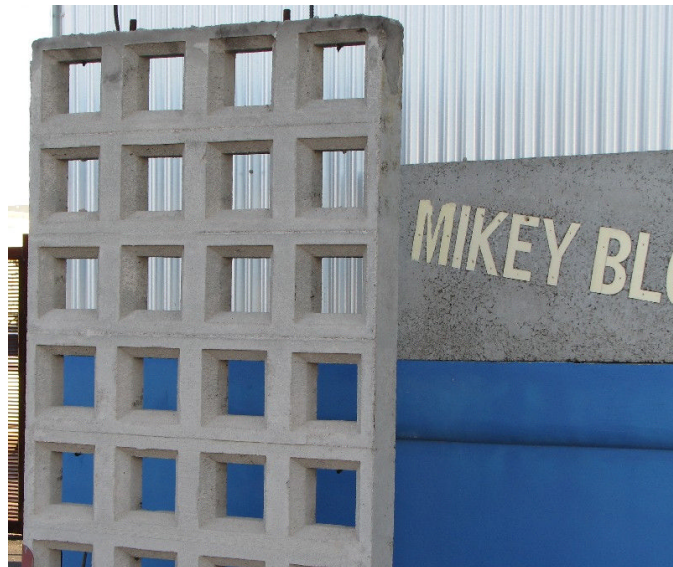
Figure 2: Mikey Block Wall Section with Foam Removed
