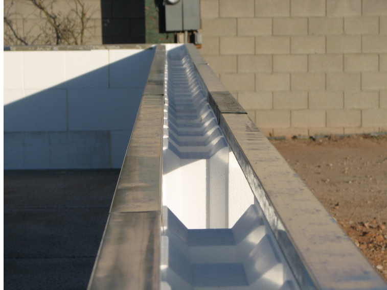
Figure 8: Using 2.5" Track to align the wall
